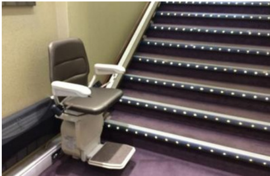
Stairlift at bottom of stairs to upper ground floor
