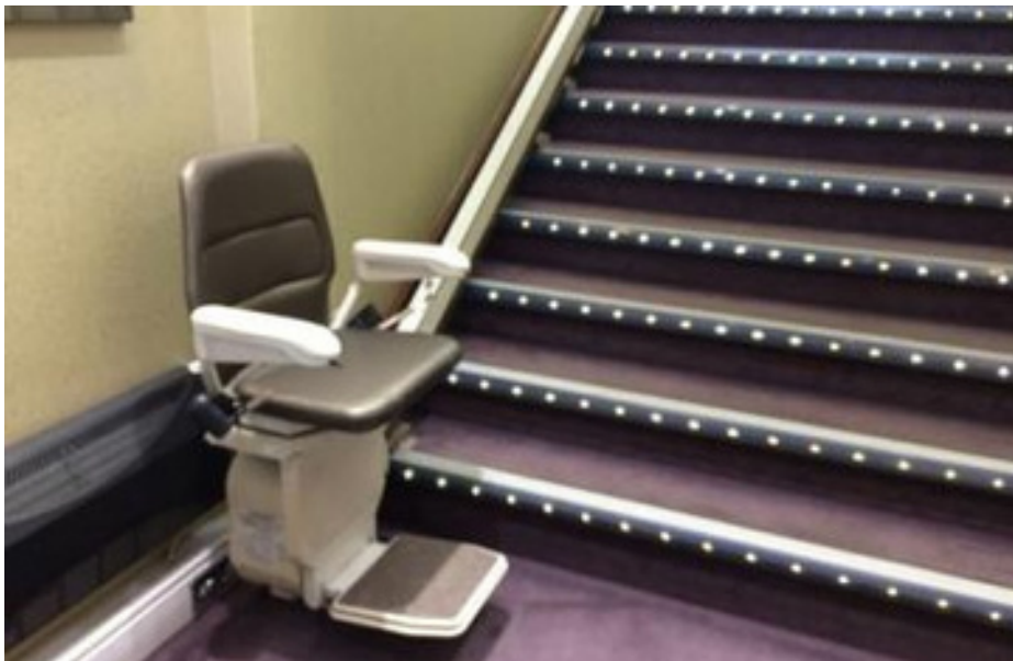
Main stairs with stairlift
