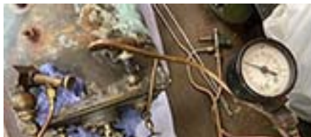
Initial pressure test on the boiler.
