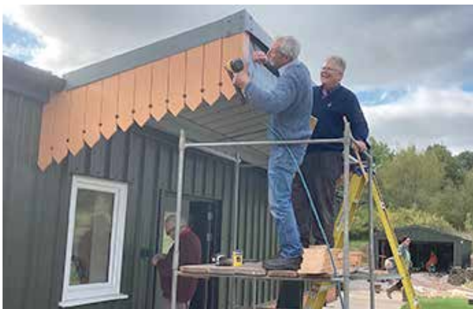
Maurice Hartnell is fixing the GWR style valance boards to the canopy on the clubhouse.
