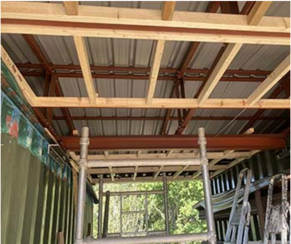
Showing the lifting beam between the two containers..
